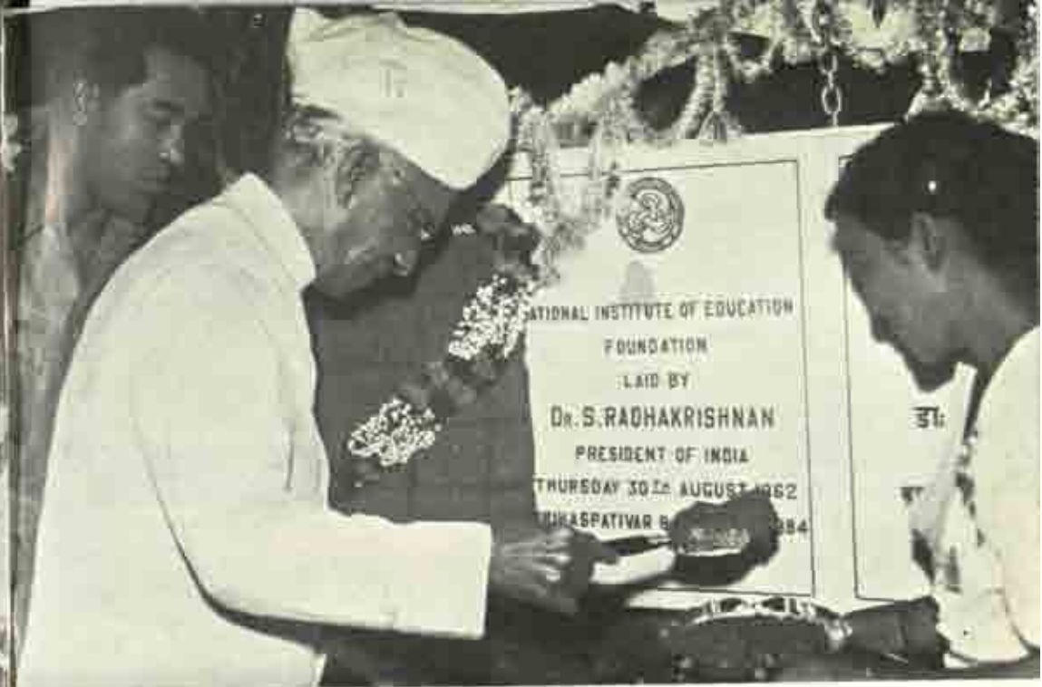
Laying the foundation-stone of the new building of the National Institute of Education at Adhchini, 30 August, 1962
